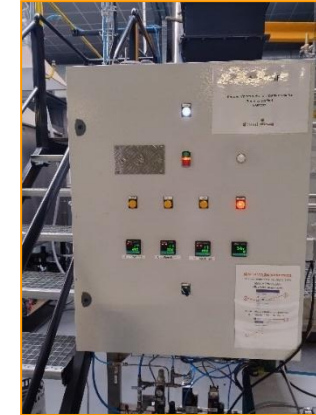
Main electrical board and datalogger unit
